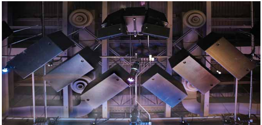
A V-shaped, end-fired line array of six OAP Audio TR 218 subwoofers flown behind the center speaker cluster helps create pattern control of the low frequencies.
