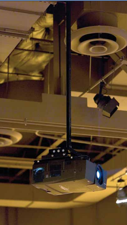
Front projection onto the dual-screen system in the new worship space is handled by two Christie Digital LX 66 6500-lumen LCD projectors.
